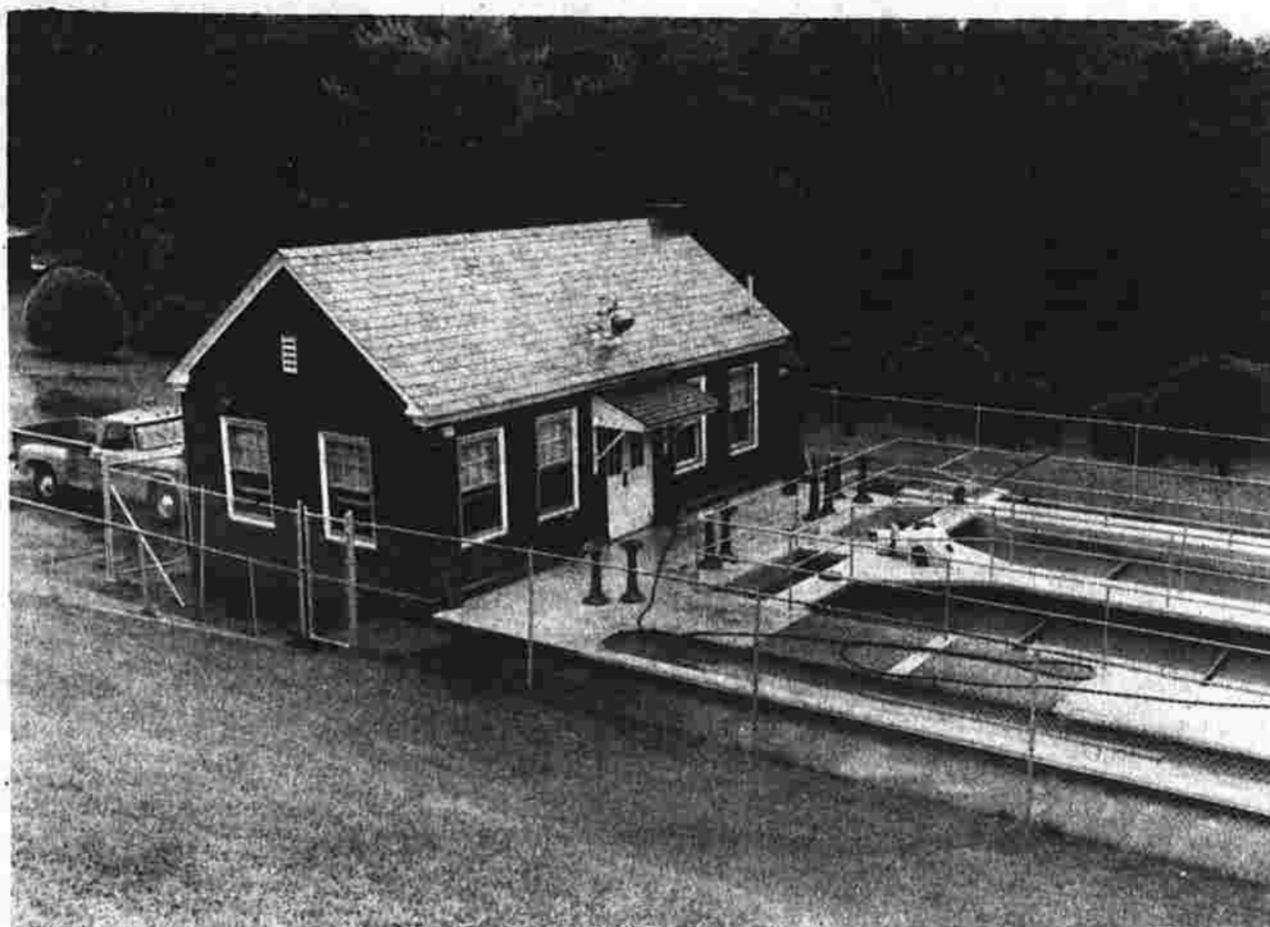
8th District sewage treatment plant opened in 1938.
